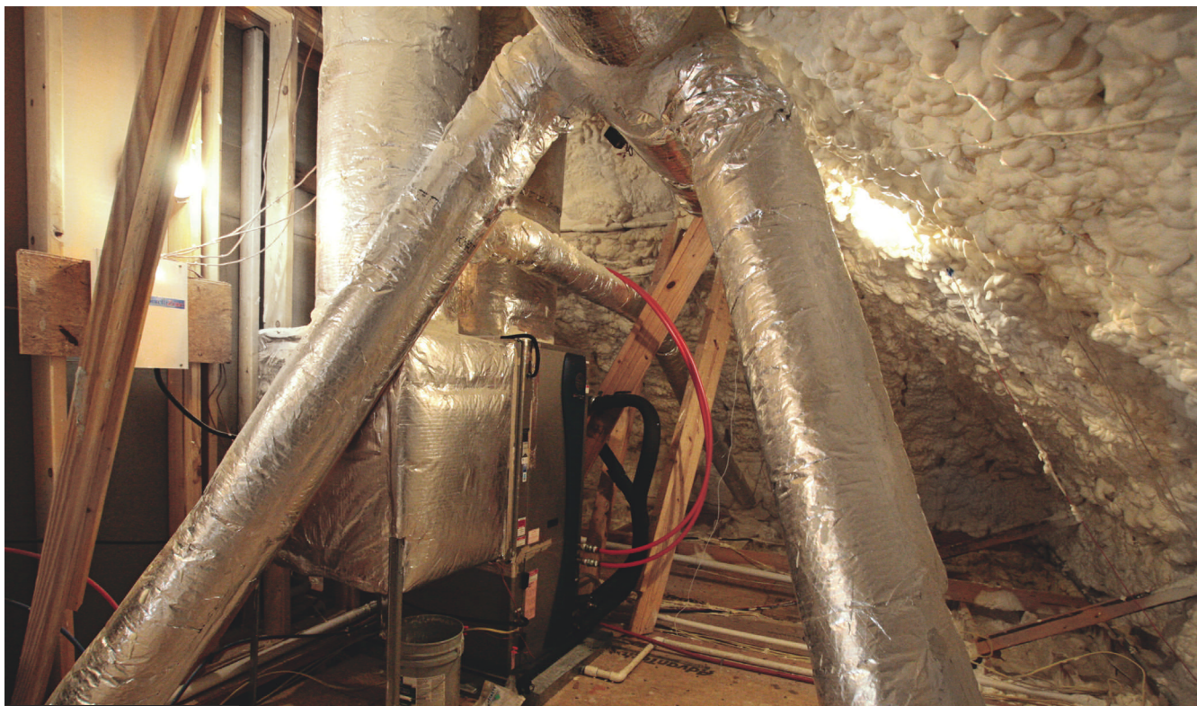
GEOHERMAL EQUIPMENT was installed in the air-conditioned, insulated attic (above).
